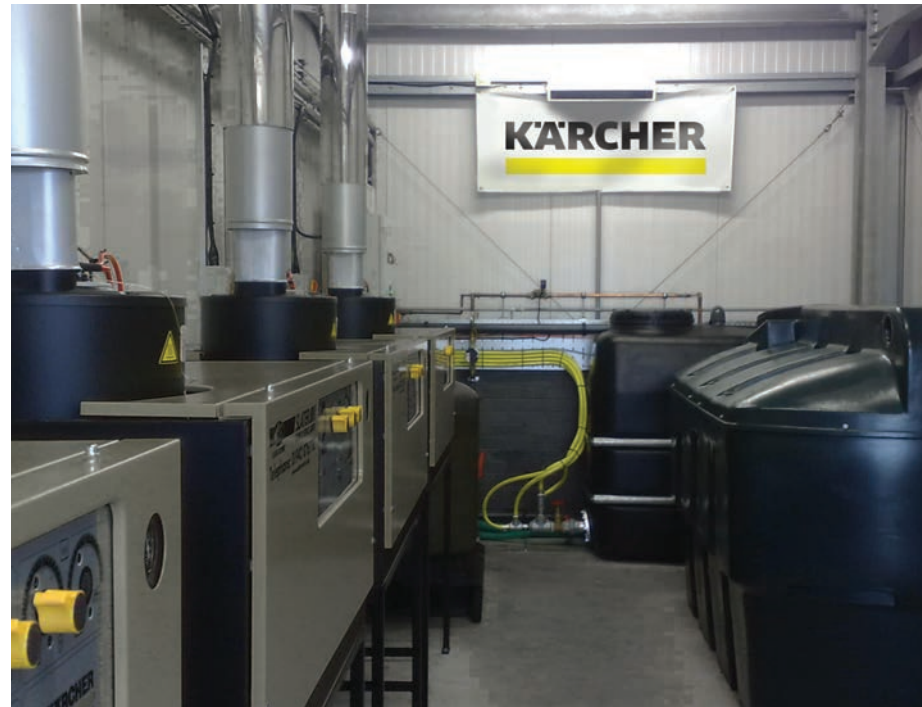
EXAMPLE OF 4 BAY PLANT ROOM INSTALLATION WITH BULK FUEL, DETERGENT & WATER RECYCLING SYSTEM
